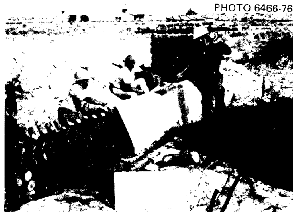
Fig. 11.7. Covering the limb-covered pole frame with bed sheets. Salt cedar limbs had first been placed crosswise over the lightly constructed pole frame.
